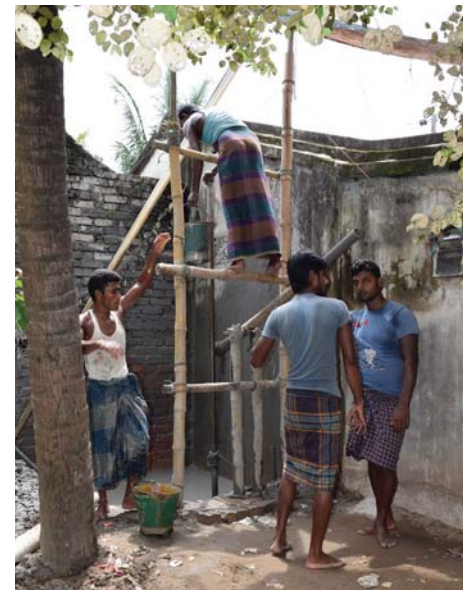
Multi-level monitoring well installation by local driller
